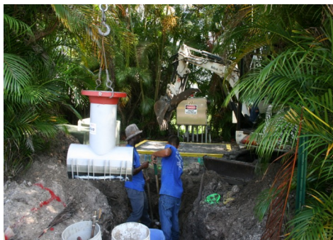
Lift Station 30 gets a new 150 pound valve and a wet well rehabilitation before the two re-built 20 hp motor and pump assemblies are installed.
